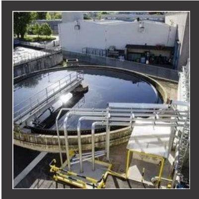
Sewage Treatment Plant
