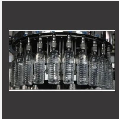
Packaged Drinking Water Plant
