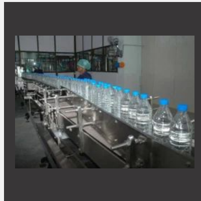
Packaged Drinking Mineral Water Plant
